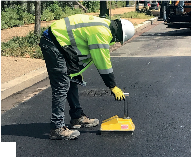
Freshly laid asphalt being measured with a density gauge based on a gamma-emitting isotope like caesium-137.
