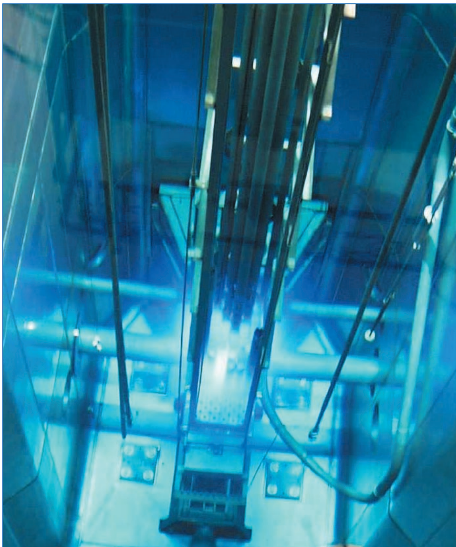
A 'swimming pool' research reactor at the Institute for Nuclear Technology in Portugal. The blue glow (Čerenkov radiation) arises when radiation passes through water, which is used to slow down (moderate) the neutrons formed in fission so they are able to cause other uranium nuclei to undergo fission. Reactors like this have many industrial and scientific uses. (Courtesy the Institute for Nuclear Technology, Lisbon, Portugal.)
